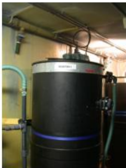
Fig. 11. Denitrifying bioreactor with suspended carrier (R1)
