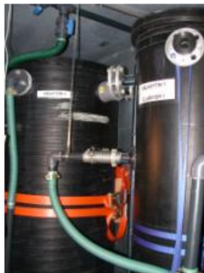
Fig. 12. Moving bed aerobic bioreactor (R4) and clarifier (C1)
